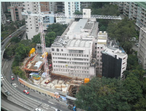
Elevation view of the construction site of the Main Building
